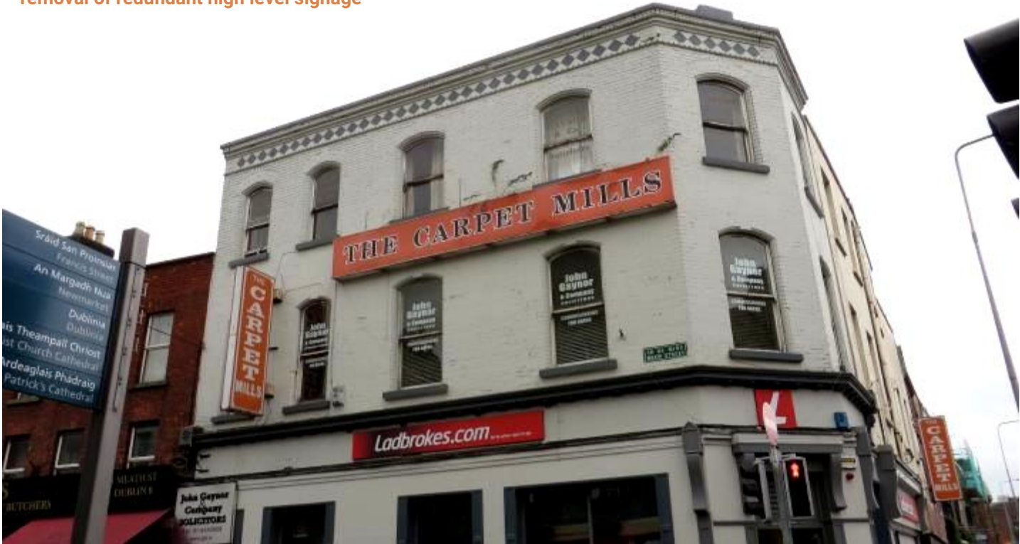
Before and after image of No 46 Thomas Street with removal of redundant high level signage
