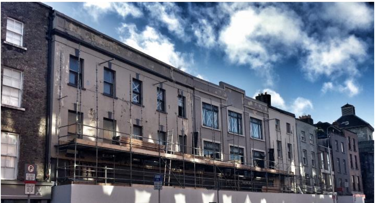
Looking to the future: terrace on Thomas Street undergoing renewal
