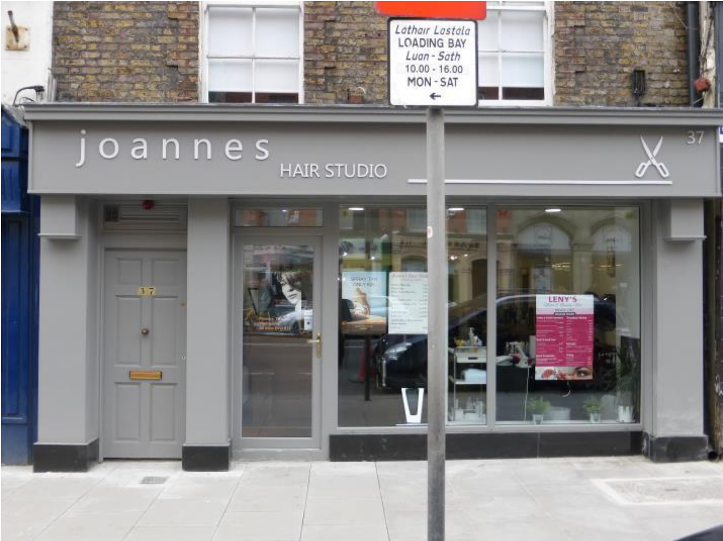
Before and after images of No 37 Thomas Street with work undertaken with the support of the Shopfront Improvement Scheme. Design detail by Damien Culligan Architect for the applicant.
